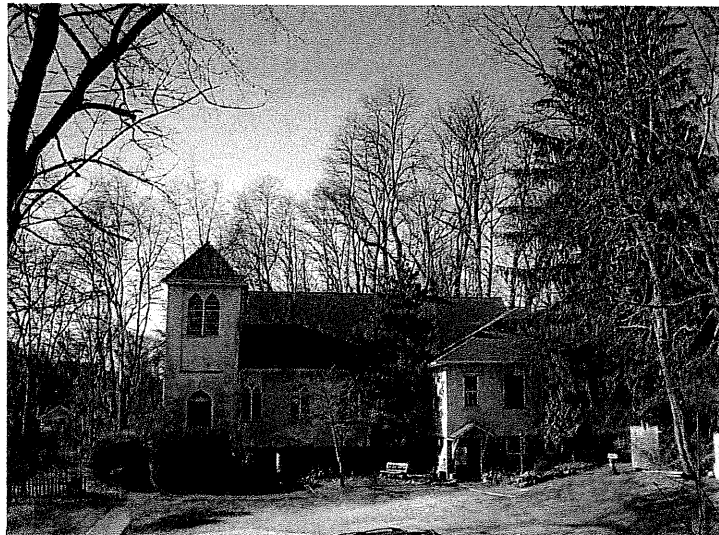
The existing chapel on the left and the social space on the right. Parking on site is in the foreground.
